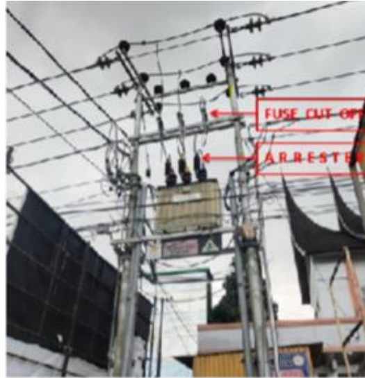
FIGURE 5. Portal Substation Construction After Changes to Arrester Installation Analysis After Fuse Cut Out (FCO) ULP Bukittinggi (GD 541/PLNUP3PYK/160KVA)
